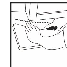
Trim door frames by placing a plank upside down next to the frame and cutting to the necessary height.
